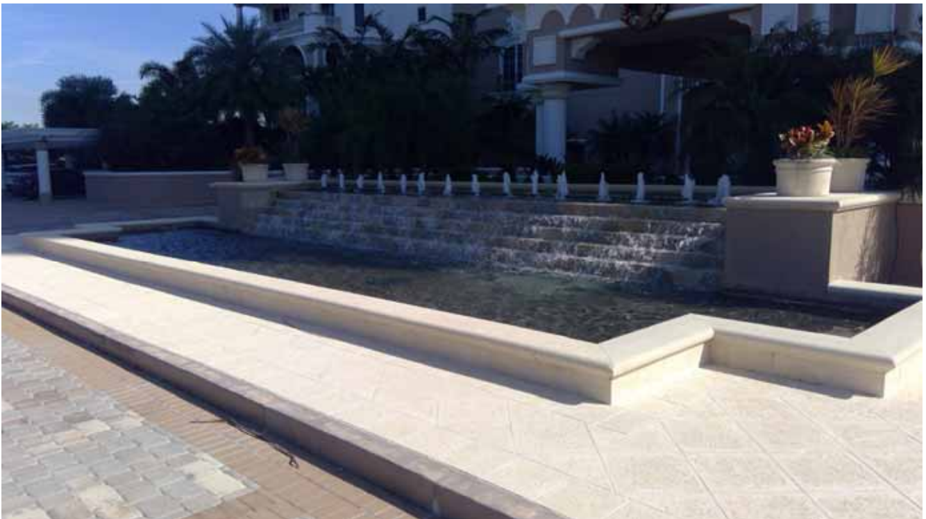
Water Feature - Arrival Deck
