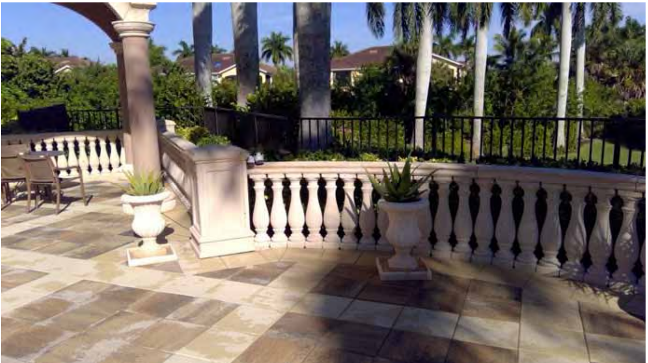
Fence & Railing - Pool Deck
