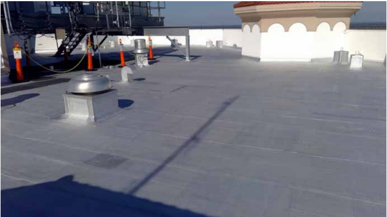
Tower Roof - Modified Bitumen
