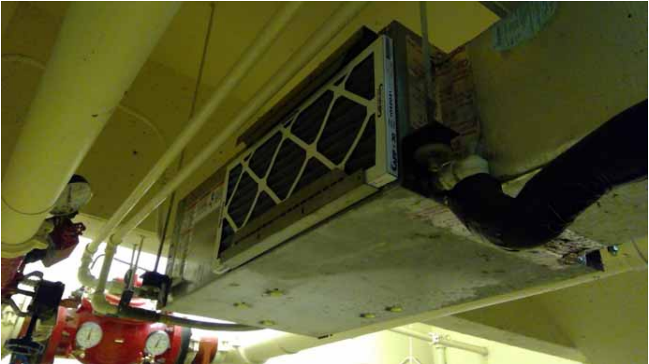
A/C Trash Room - North
