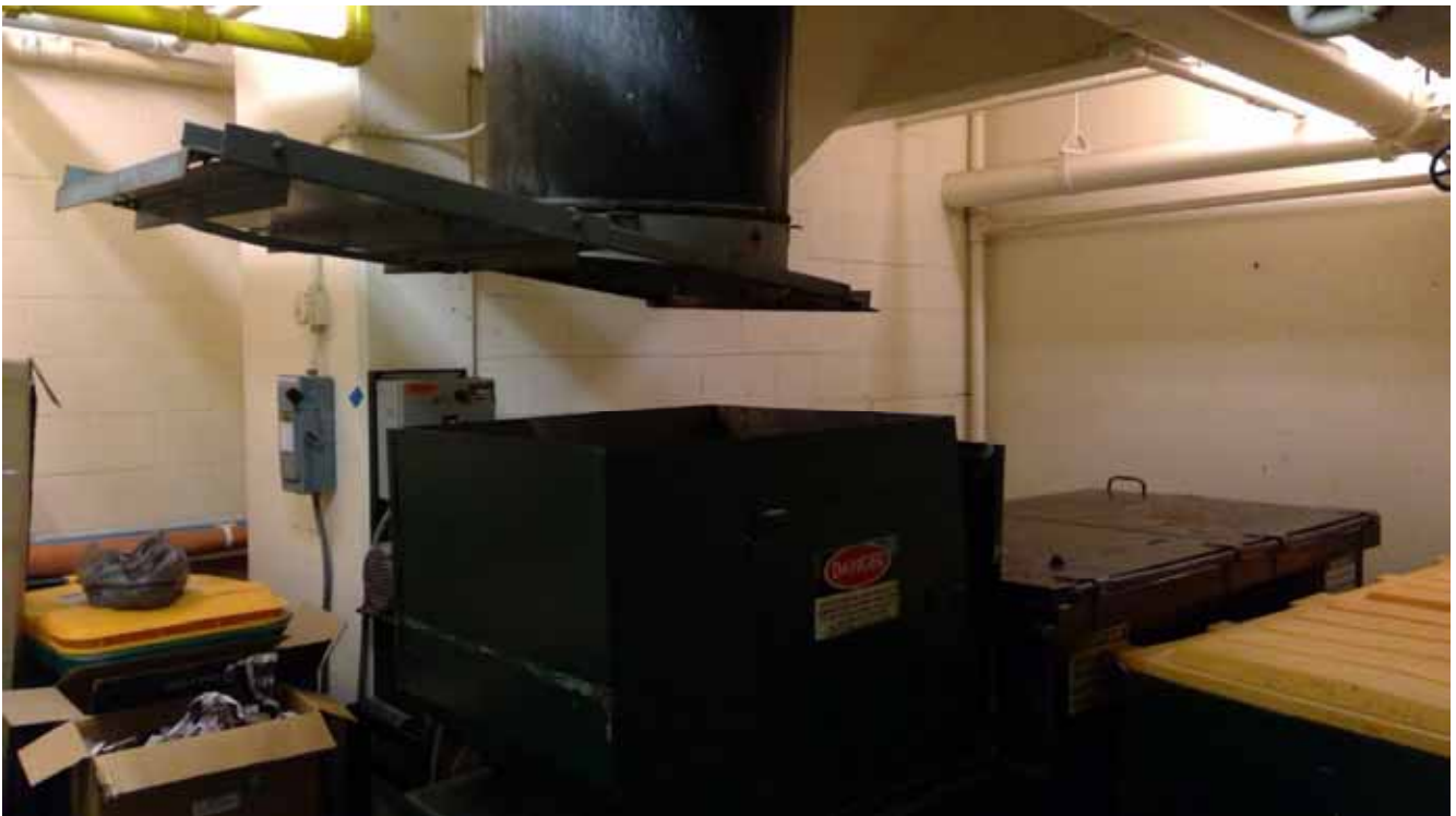
Trash Chute - South
