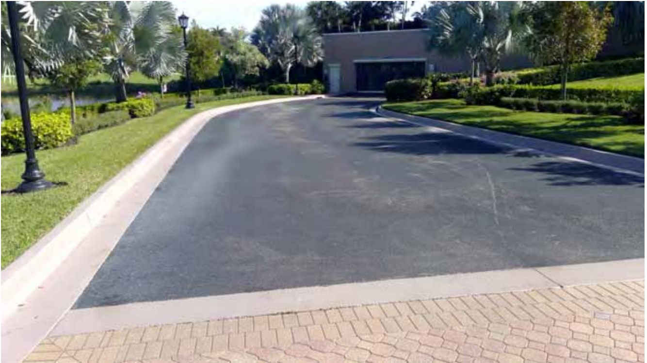
Asphalt Driveway - Resident Gate
