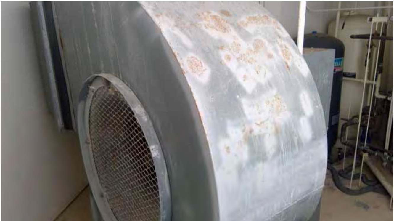
Stairwell Pressurization - North
