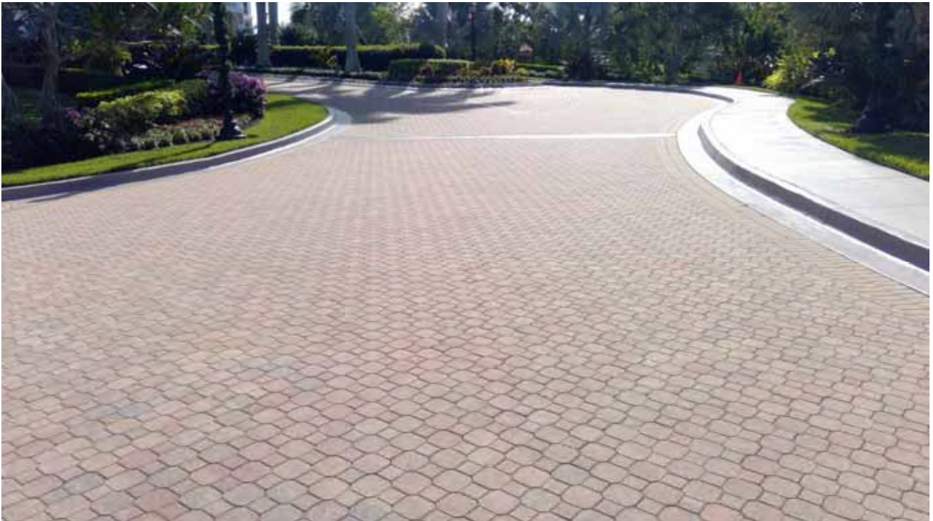
Pavers - Main Entry Drive
