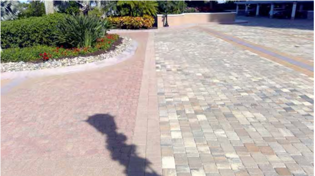
Pavers - Arrival Deck
