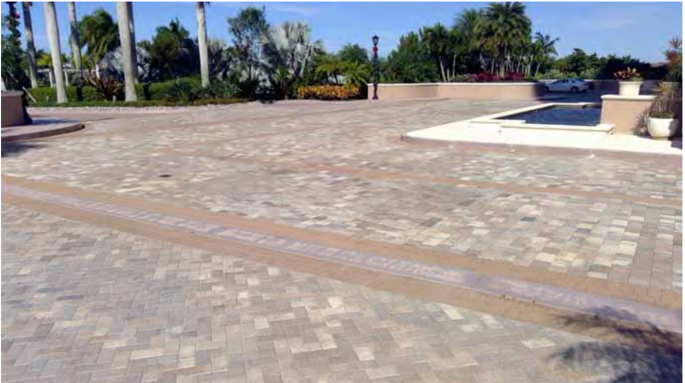
Pavers - Arrival Deck
