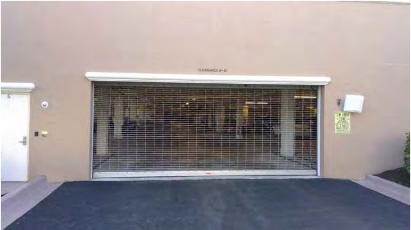
Resident Gate - Garage
