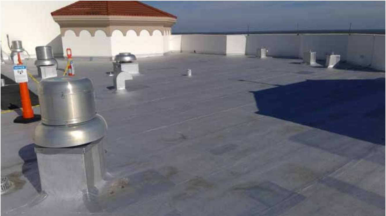
Tower Roof - Mod Bitumen
