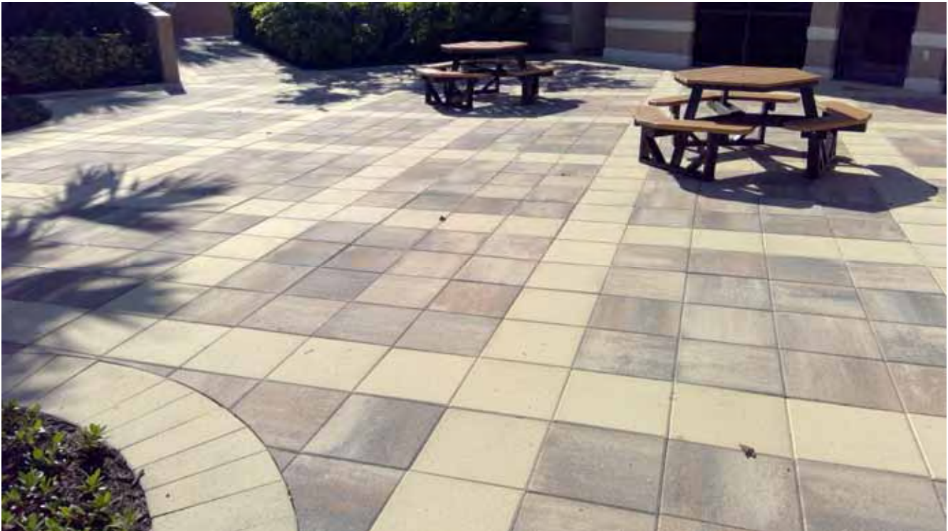
Paver Deck - Pool Building
